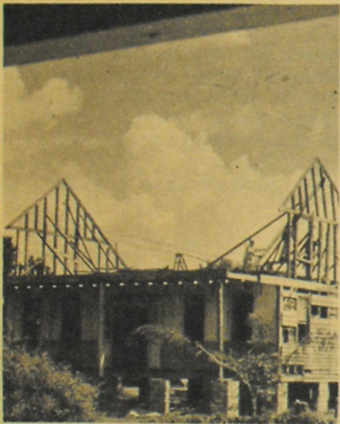
In preparation for move, roof of cottage was folded flat before structure was loaded onto flatbed truck
